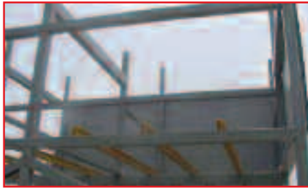
Cooling tower structure of pultruded FRP shapes
