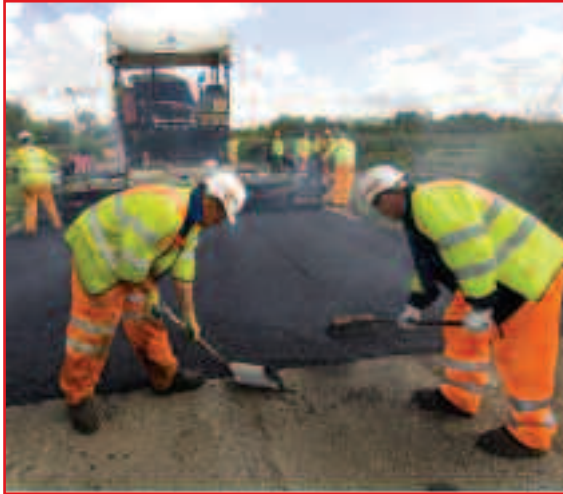
Road re-surfacing project in Northall, Buckinghamshire
