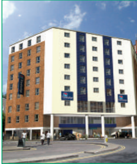
Uxbridge Travelodge Hotel – complete building
