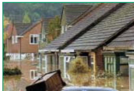
Flooding in an urban environment
