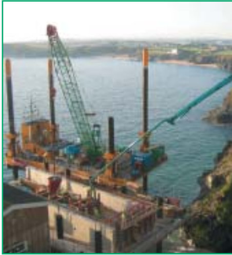
Engineering work in the coastal zone.
