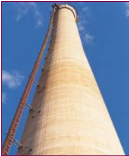
(Top) Quick and efficient construction with pre-cast elements (Courtesy of The Concrete Society) (Above) In-situ slipformed concrete tower; an alternative to the precast option (Courtesy of Bierrum)
