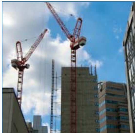
Tower cranes are in common use in construction
