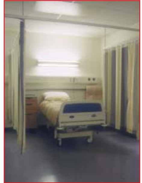
A combination of uplighting and downlighting can give a bright environment with enough light for patients to read.
