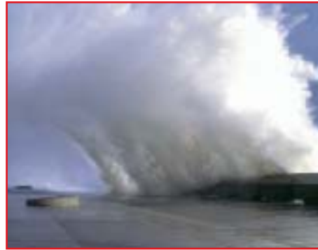
Severe wave overtopping at the Samphire Hoe seawall. (Courtesy of Eurotunnel and The White Cliffs Countryside Project)
