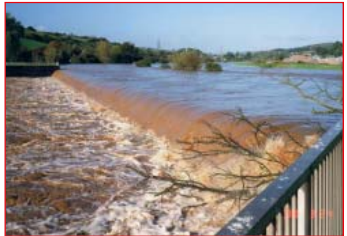
(Top) River Exe side weir with no flow and (Above) in flood
