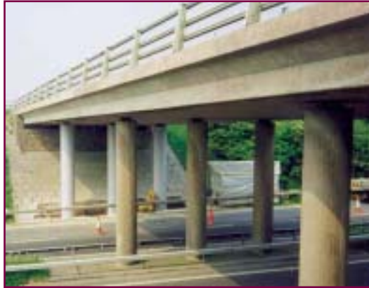
Bible Christian Bridge, Cornwall: columns strengthened with FRP
