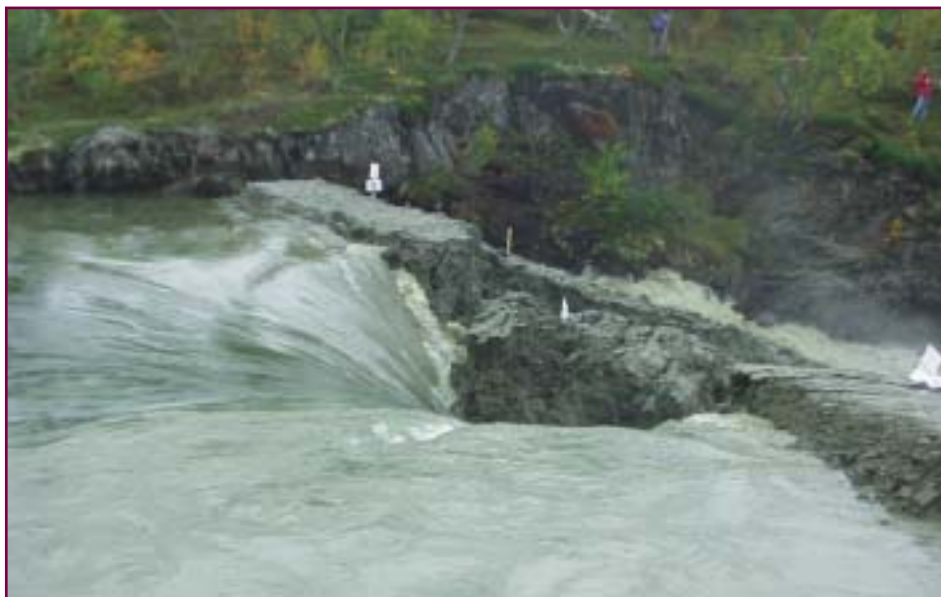
Breaching a 6m high clay embankment in Norway (Oct. 2002)
