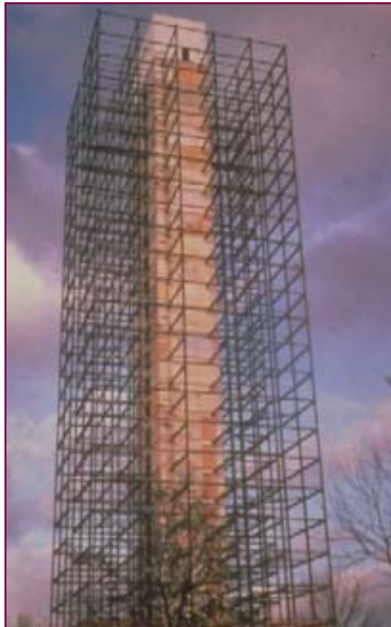
Winterton House, London – stripped to its steel structure prior to refurbishment
