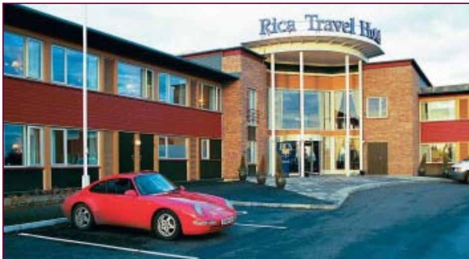
Example of timber structure – prefabricated modular units – where vibrational and acoustic performance control serviceability design. Courtesy C. J. Mettem, TRADA Technology.
