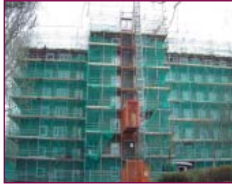
Glazing replacement contract
