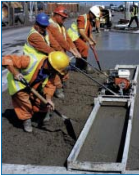
Construction of trial access road using non-ferrous industry waste as aggregate
